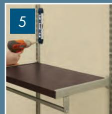
Once all shelves are installed, level, mark and secure each hole of the left standard to the wall.
