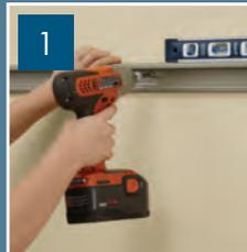
Level and secure hang track. Fasten each hole.
