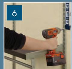
Level and secure all holes of the right standard to the wall.
